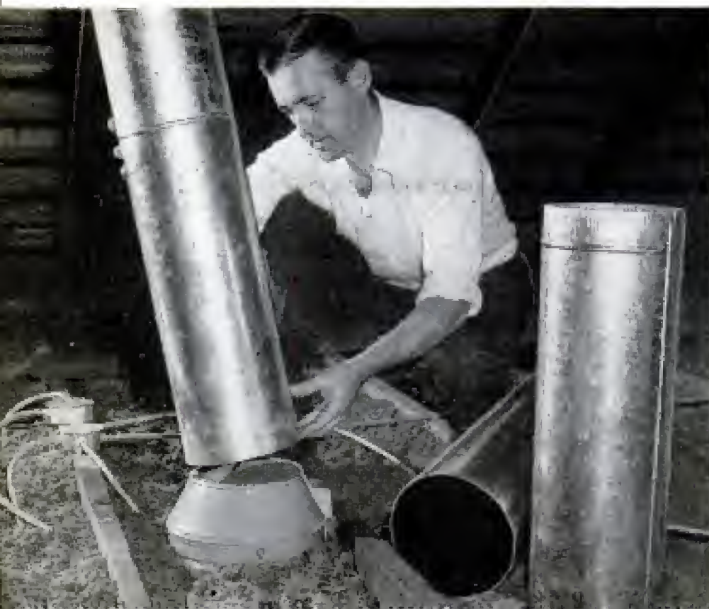
Below, reducer capping top of housing takes standard 8-in. furnace pipe to vent fan through roof as in drawing at right. The reducer has back-draft damper
